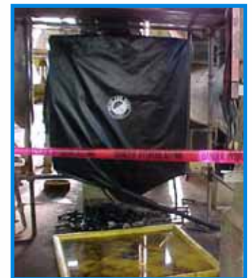
Containment of Contaminated Hydroblast Water
