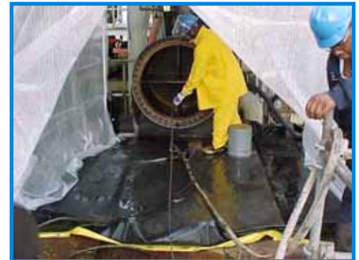
Containment of Contaminated Hydroblast Water
